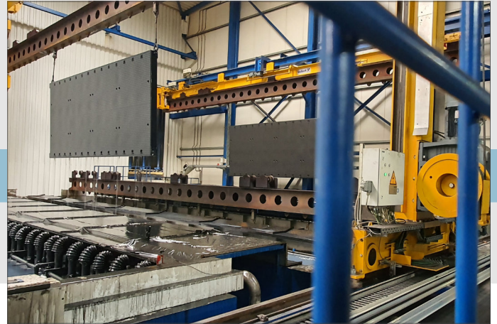
Goods carriers move the huge truck loading bridges through the cathodic dip coating line
