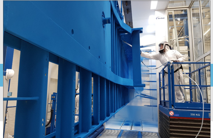
Areas inaccessible to the automatic guns are manually coated
